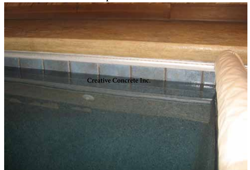
Auto-covers provide safety, debris protection and aid in temperature control.
